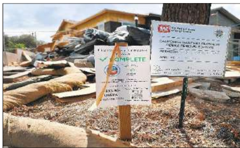
THE LEAD in Altadena's soil is thought to come from burned lead paint, which can damage the brain. ALLEN J. SCHABEN LOS ANGELES TIMES
